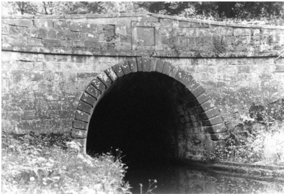
Eastern Portal of Berwick Tunnel - see back page
