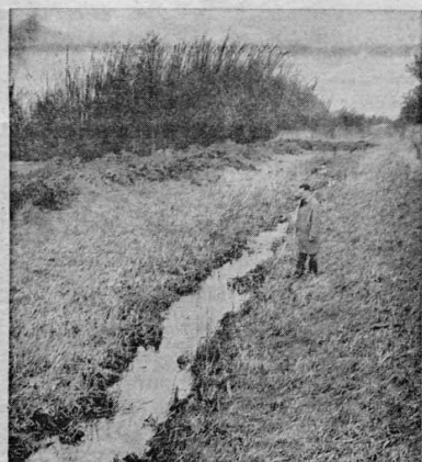
THE CANAL BED before reclamation. The soil from the left-hand bank has been removed for filling in higher up the canal.
