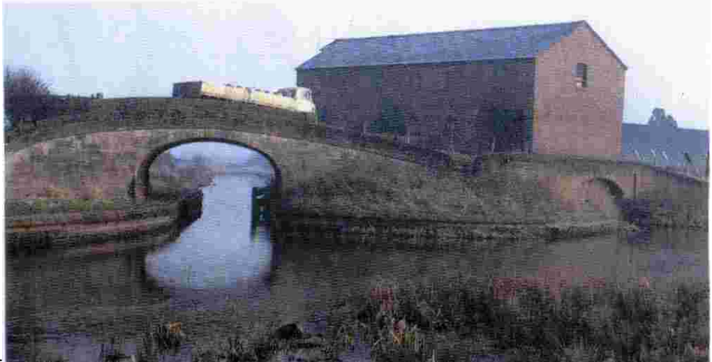
Wappenshall Junction with the Newport Branch passing under the bridge. The bridge to the right allowed boats to unload directly into the warehouse, which still stands today.
