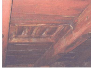
First floor pulley wheel. Note the wooden hand operated brake.
